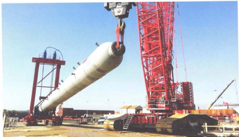
Two reactors were transported, lifted and installed in a refinery in the north of Italy by Fagioli in March. Each reactor was more than 45 m long, with a net weight of almost 400 tonnes. Fagioli used 30-axle line SPMTs to move the reactors, then a crawler crane LR1750 with a capacity up to 750 tonnes, and a tailor-made tailing frame structure positioned on 2 x 10-axle line SPMTs, with two L600 strand jacks on top of the structure used to perform the tailing operations.
